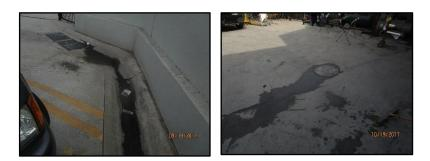
Location: Auto shop on Alondra Avenue. Non-compliance (9/19/17): Discharge from an auto-washing station is entering a storm drain. Follow-up inspection (10/19/17): Auto-washing station was moved, and the wash
